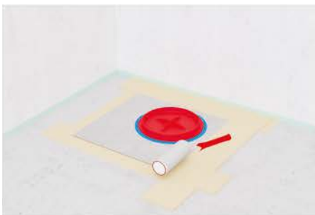
10. Apply moisture proofing compound
