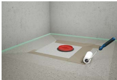
8. Apply waterproofing in the whole shower area and on (and under) the sealing kit, seal the edges with sealing tapes.
