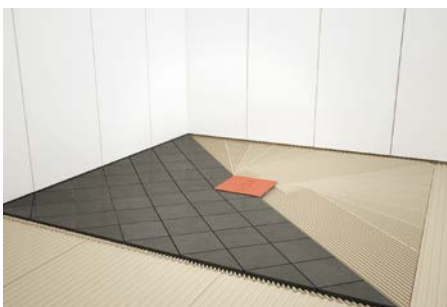
10. Adjust the extension by turning to the tile layout (360° turnable), lay the tiles.
