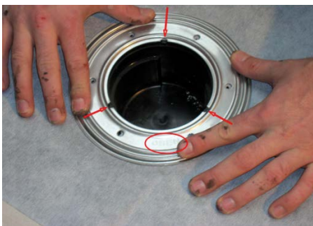
4. Apply the waterproofing membrane
