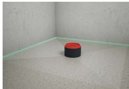
5. Insert floor screed and create a slope to the drain by minimum 2%.
